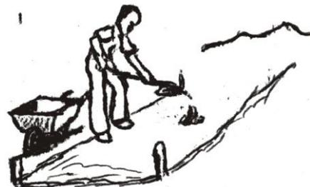
3. Dig a narrow trench, about 30 cm (1 foot) wide and about 30 cm (1 foot) deep (generally until you can see the subsoil). Set aside the topsoil you have dug out; you will need it later.
